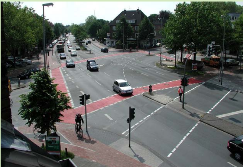
An intersection with adequate crosswalks, traffic calming measures, textured bike-ways, pedestrian and cycling oriented traffic lighting, and pedestrian islands.
