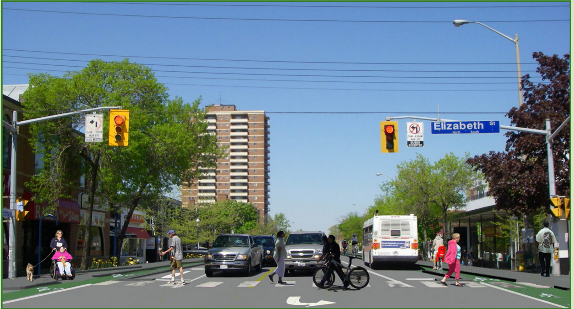
Left-turn centre lane with on street parking, widened sidewalks, physically separated bikelanes, bus stops, and car parking on north side.
