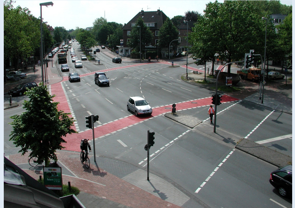
An intersection with adequate crosswalks, traffic calming measures, textured bikeways, pedestrian and cycling oriented traffic lighting, and pedestrian islands.
