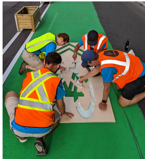
Volunteers paint bike lanes along Danforth Ave.
